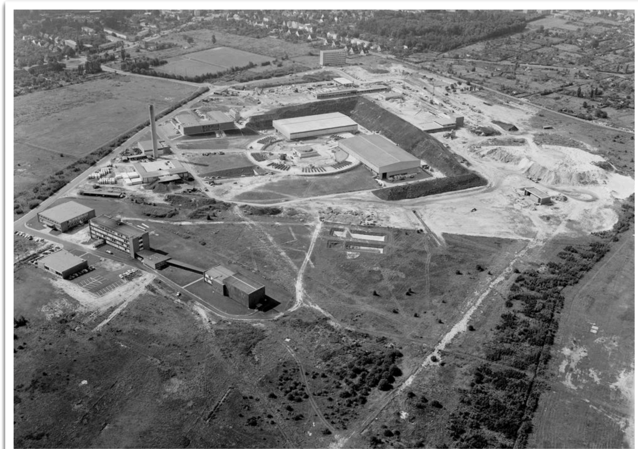
Construction of the DESY Synchrotron, 1961
