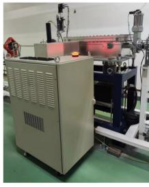
Figure 9: Kicker magnet and its high stability pulsed power supply installed in the undulator tunnel.
