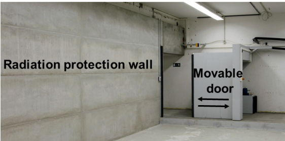
Figure 2: The radiation protection wall and the movable door in the tunnel annex.
