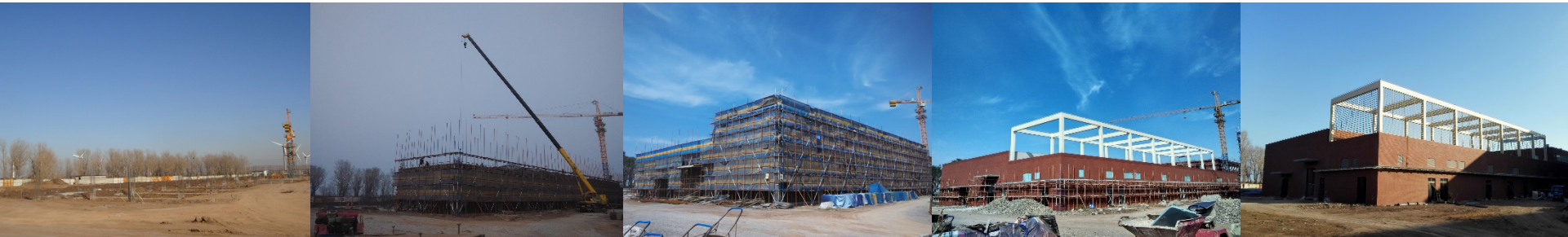
2014.11- 2016.01 DCLS Building construction
