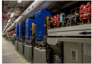
Figure 1: First bunch compression chicane.
