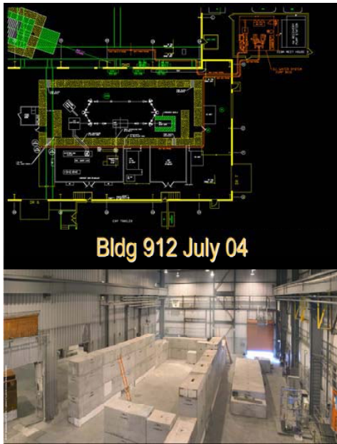
Fig.3 The layout of the facility (top) and the photograph of the shielded vault for R&D ERL under construction in the bay of Bldg. 912. The bay is equipped with an overhead crane. The control room is located outside of the bay in a separate building.
