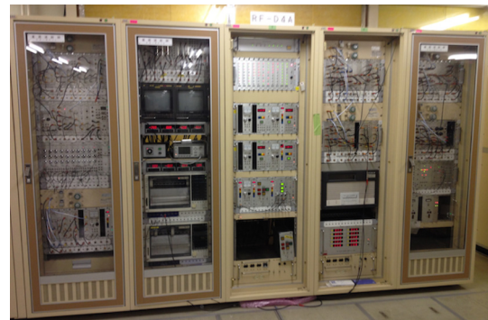
Figure 7: Old LLRF control system, which was used in KEKB operation, continues in use for SuperKEKB.
