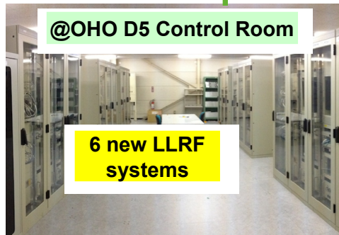
Figure 6: Installation appearance of the new LLRF control systems in the RF control rooms at D4 (upper) and D5 (lower) section.
