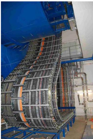
Figure 6: Flexible cable tray.
