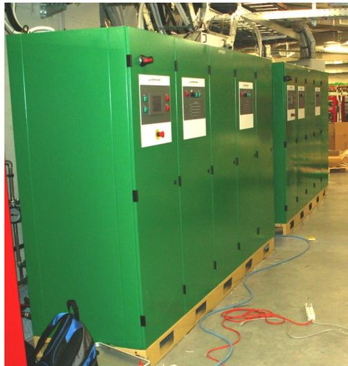
Figure 3: Dipole Converters' Cabinets.
