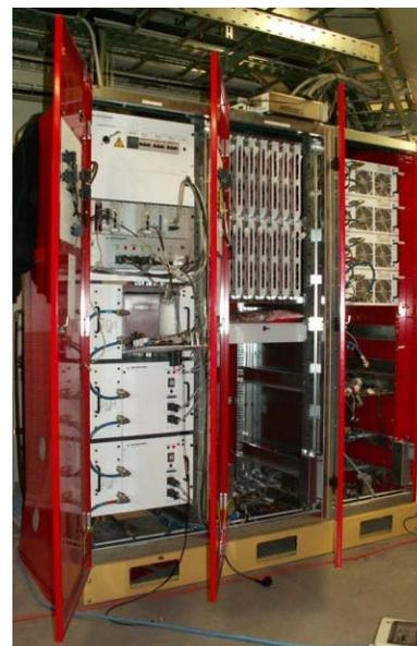
Figure 4: Quadrupole Converters' Cabinet during the installation phase.
