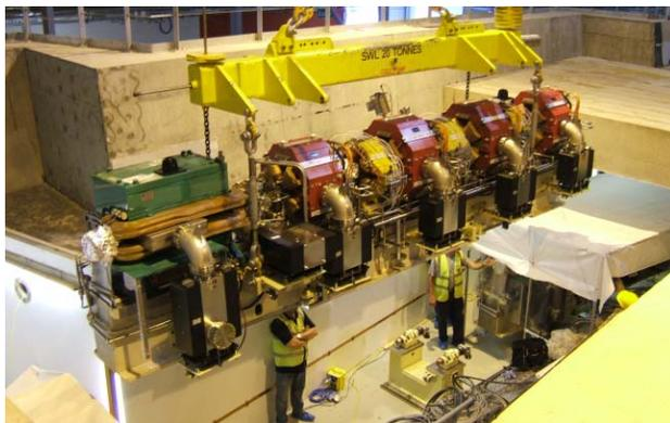
Figure 2: Installation of a girder in the storage ring.
