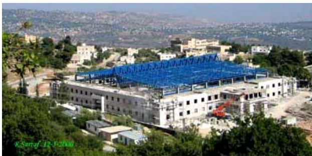
Figure 1: A panoramic view of SESAME building during construction (May 2006).
