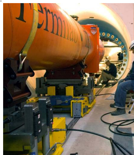
Figure 4: Q1 is moved with the motorised bogies into the ATLAS experimental radiation shielding
