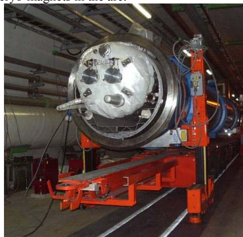
Figure 3: MUE assembled around a magnet lifted off the trailer
