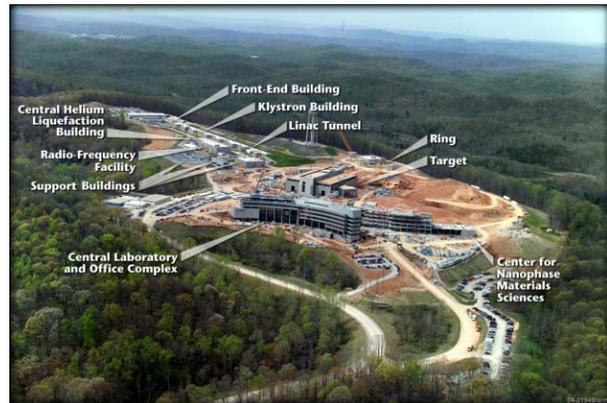
Figure 1: The photograph shows the SNS site with the finished accelerator facilities in the upper left and the Target building, Central Laboratory Office and the Center for Nanophase Material sciences in the foreground.
