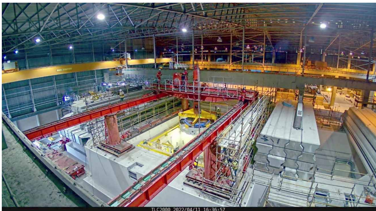
Figure 4: Rigging of the magnet yokes into the centre vault.
