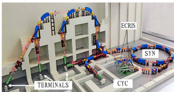
Figure 1: Layout of HIMM. ECRIS: ECR ion sources. CYC: Injector cyclotron. SYN: Synchrotron. TERMINALS: Treatment terminals.
