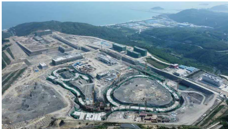
Figure 2: Civil construction of the HIAF project.
