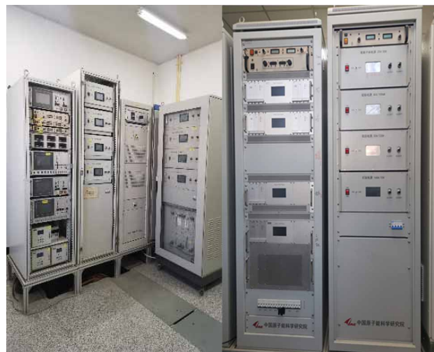
Figure 1: Power supply integration comparison (Left: discrete power supply for CYCIAE - CRM, Right: integrated power supply for CYCIAE-14A).
