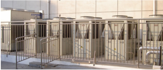
Figure 4: The picture of cooling tower and cryogenerators.
