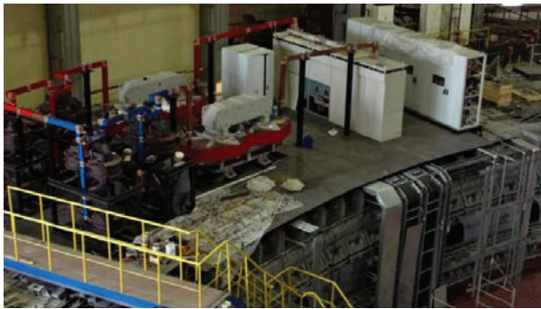
Figure 3: Power supplies of the Booster magnets mounted on the top the yoke.
