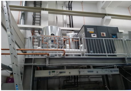
Figure 1: Compressor system for driving up to three turbines at HIM. Size of compressor (grey box, upper right) is about 2,5*2*1m.
