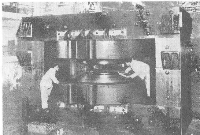
Fig.20 The magnet of the INS 63 inch cyclotron, before mounting the vacuum chamber, 1956.
