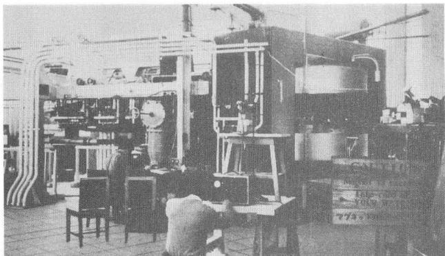
Fig.16 The Kyoto 41 inch cyclotron, completed in 1955 and afterward improved in 1973
