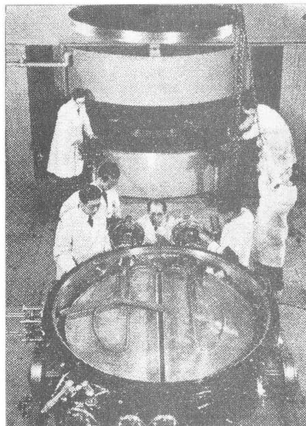
Fig.4 The old accelerating chamber for the 60 inch cyclotron, simply enlarged from the small cyclotron. In the background is seen the 60 inch cyclotron magnet.
