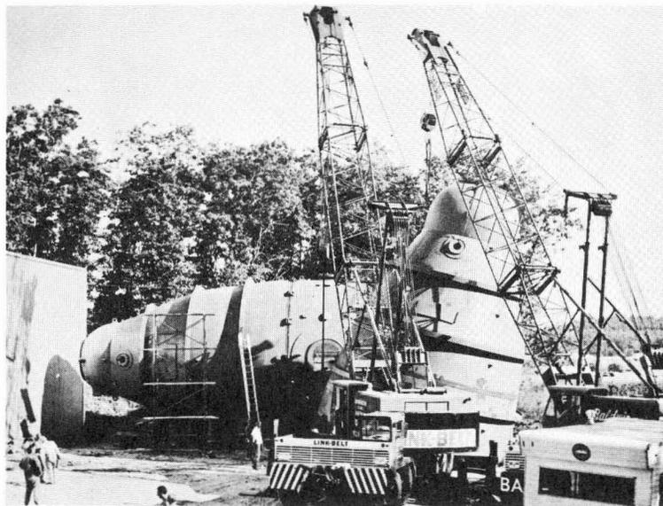
Fig. 12. A photograph of the installation of the giant pressure vessel for the TU tandem during installation at Burlington, Massachusetts
