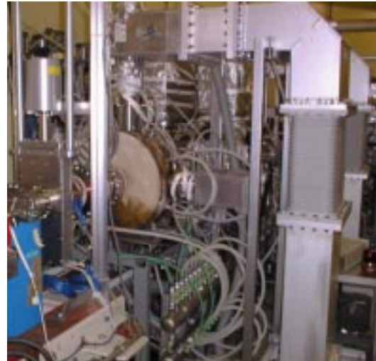
Fig. 2 New damped cavities installed in the ring.
