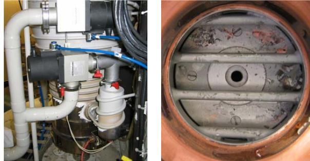
Figure 2: LHS shows Cyclone30 ISIS diffusion pump. RHS shows ion source with hydro-carbon debris.
