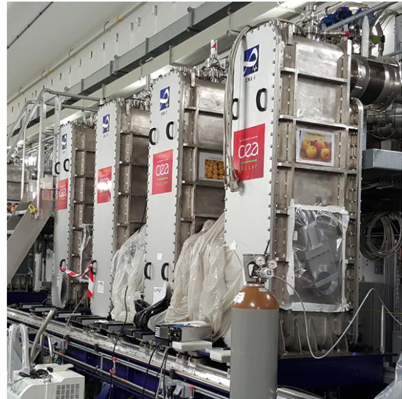
Figure 10: Low beta cryomodules installed on LINAC.
