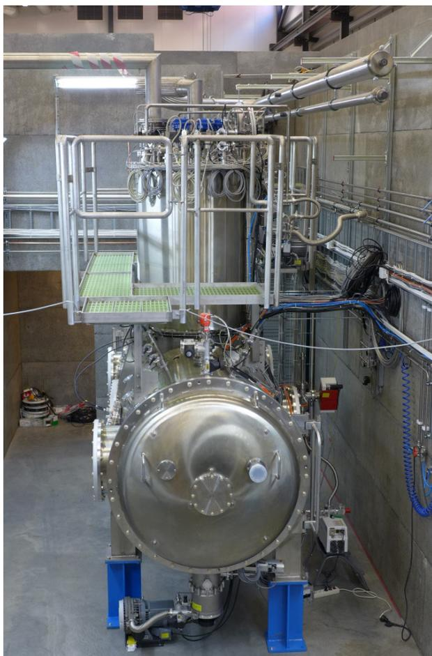
Figure 2: The HNOSS horizontal cryostat and valve box.
