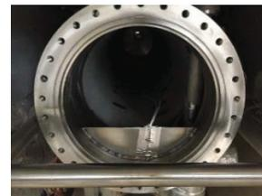
Figure 7: Liquid baffle plate welded in gas return pipe.
