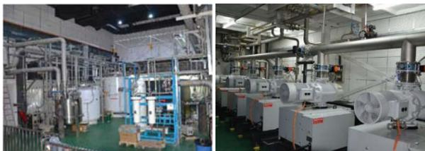
Figure 9: 2 K cryogenic system.
