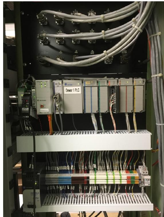
Figure 3: Dewar control PLC and I/O.
