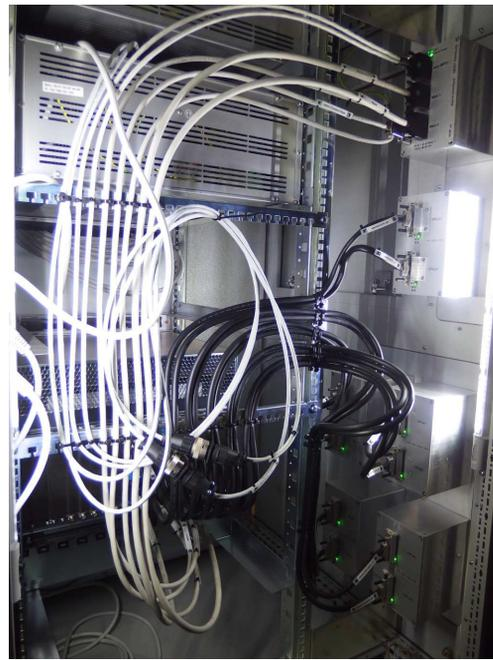
Figure 5: Rack rear view, from top: Alarm-IF, cryo/vacuum, 4x4 coupler.
