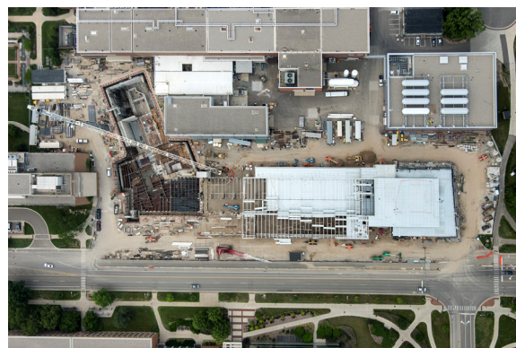
Figure 1: FRIB conventional facility construction status on August 2015.
