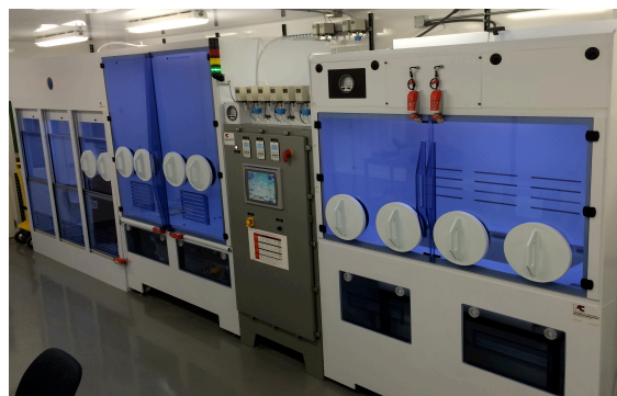
Figure 1: FRIB production chemical etching facility.
