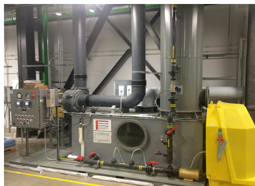
Figure 2: Toxic gas scrubber unit.
