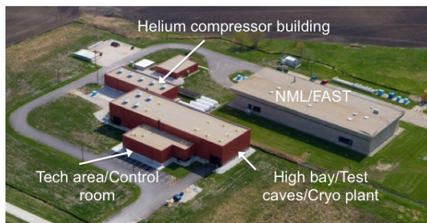
Figure 1: CMTF building adjacent to NML.
