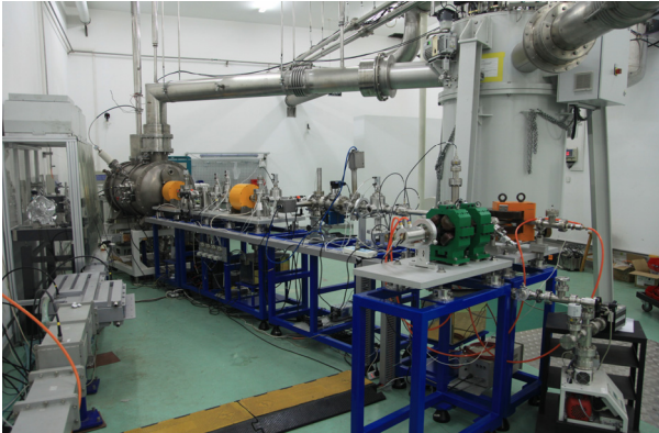
Fig. 2: New beam line for beam test of 3.5-cell DC-SRF injector.
