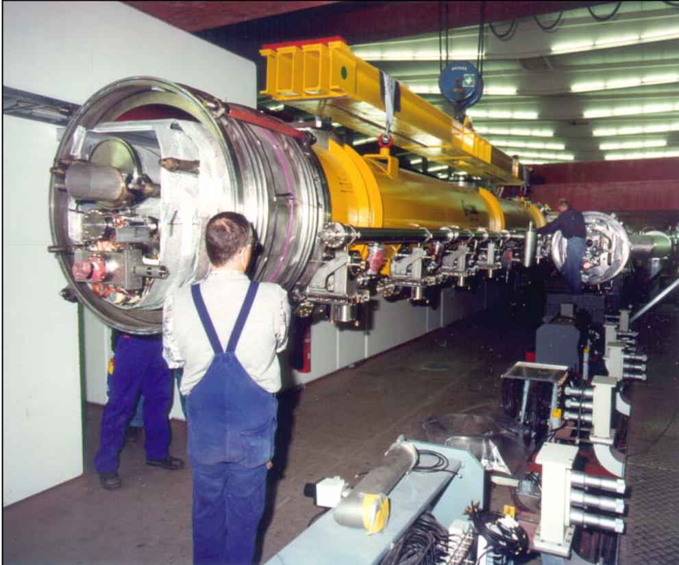
Installation of modules into the TTF linac
