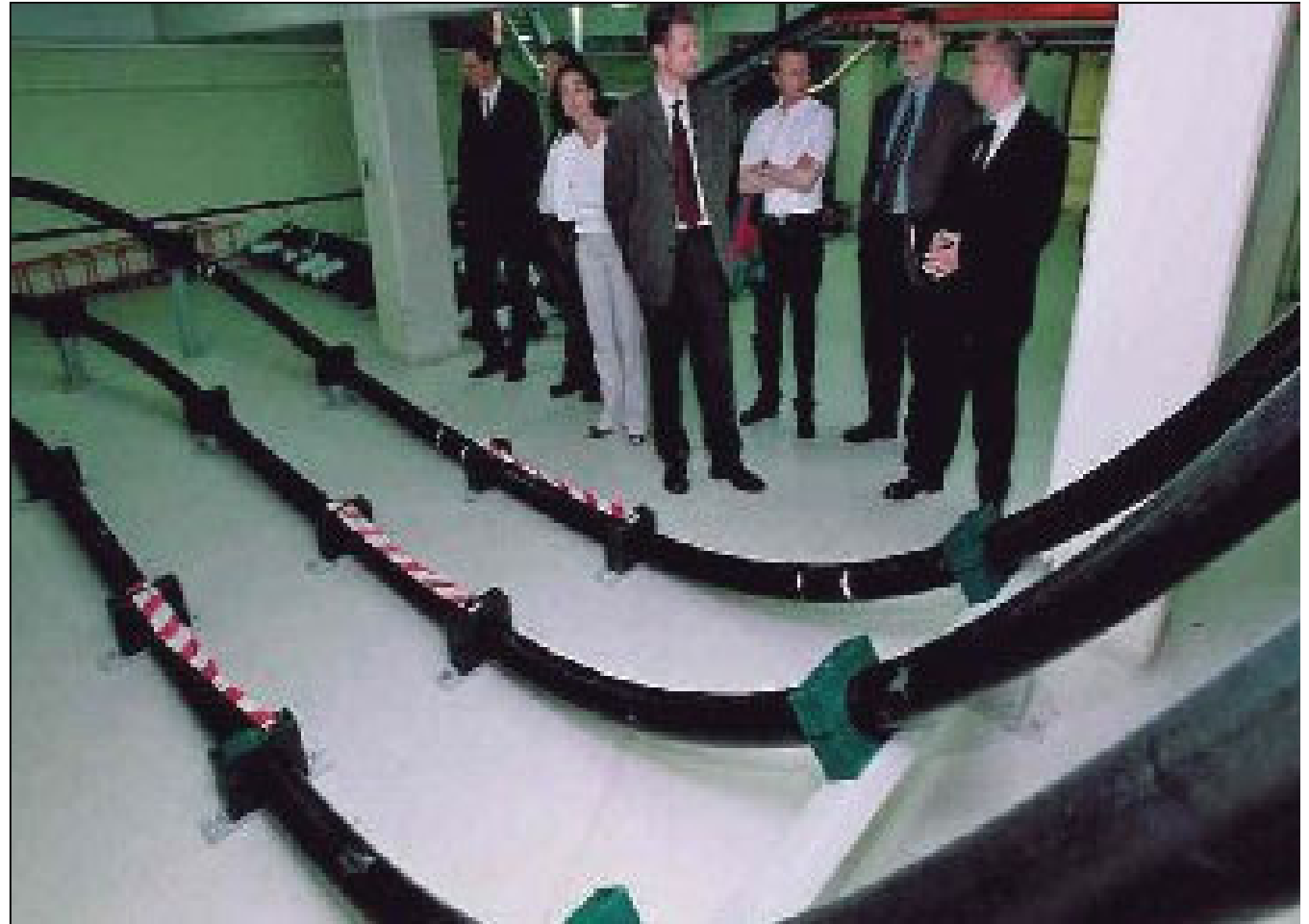
DTU-NST cable installed at Copenhagen Light & Power's Lyngby Station
