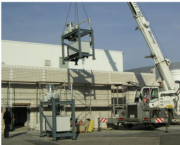
Figure 2: Linde TCF-50 Cold-box for 180 l/hr, 4.2-K LHe production (top), and Leybold vacuum pumps for 80-W, 1.8-K HoBiCaT operation being installed in the pump room (bottom).
