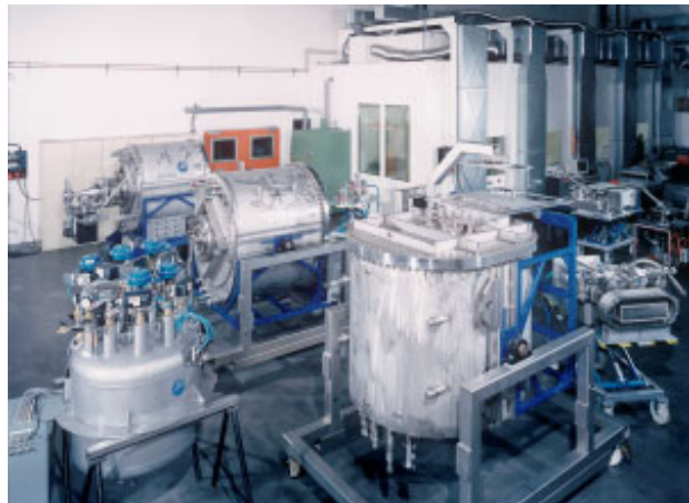
Figure 2: Assembly area of the SRF modules at ACCEL. In the upper right part the clean room class 100 can be seen where the modules need to be assembled in whenever the cavity vacuum is touched.
