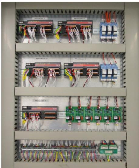
Figure 4: Typical node box layout.
