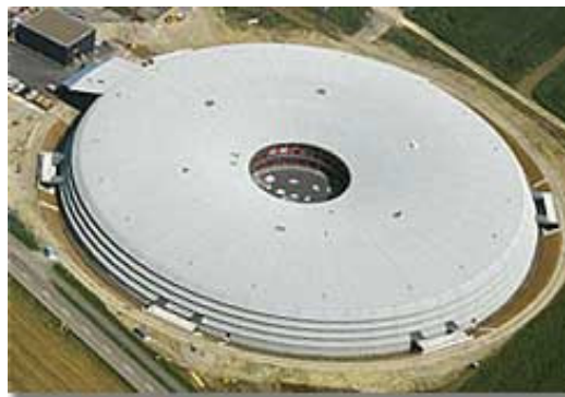
SLS (2002) 2.4 GeV \epsilon_x = 3.9 nm, \epsilon_y = 10 pm, I = 300 mA
