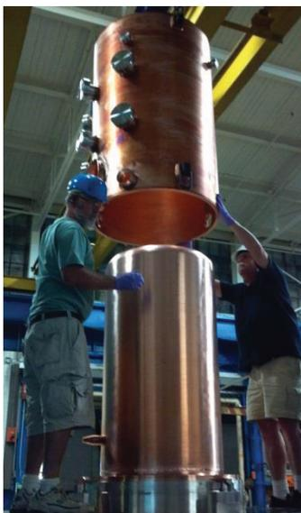
Figure 2: Positioning of outer conductor before electron beam welding.
