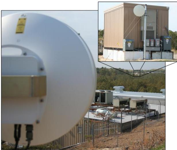
Figure 7: The microwave link transmitter for the Yellow ring, above the pickup in sector 2, is shown in the foreground. The receiver and dedicated electronics trailer, above the kicker in sector 11, are shown in the distance and the inset.
