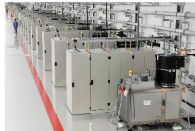
Compact modulators and klystrons For XFEL/Spring-8 (72 total)
