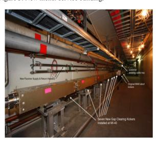
Figure 4: Kicker magnets in the Main Injector tunnel.
