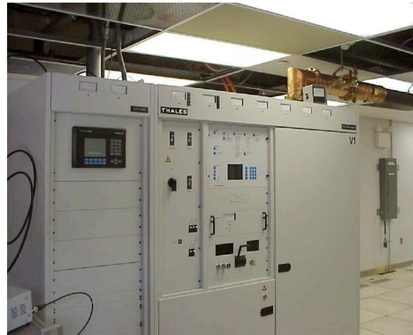
Figure 9: SRF 50 kW transmitter.
