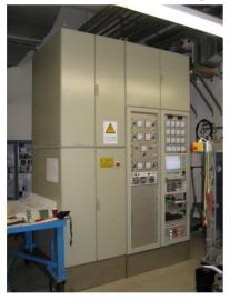
Figure 7: The supply unit with the data logging system and the low level electronics
