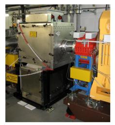
Figure 6: The cavity and power amplifier already installed in the SIS18-tunnel
