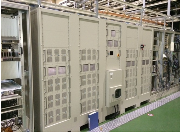
Figure 5: Photograph of a new solid-state amplifier with the output power of 120 kW.
