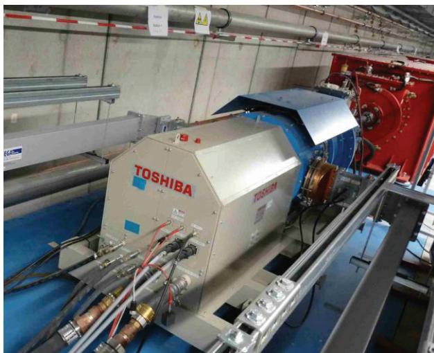
Figure 7: The first series MBK installed in the injector area of the European XFEL.
