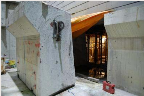
Breakthrough from ARIEL tunnel to E-hall, July 7th
