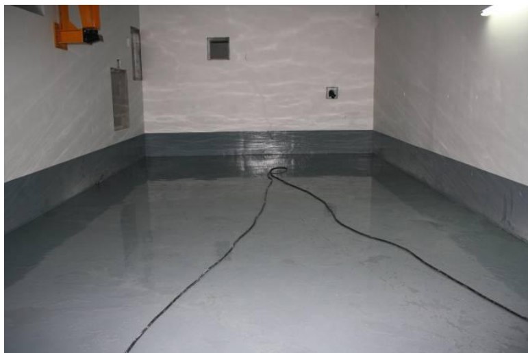
1/3 room ready to receive the ECR source and LEBT1
