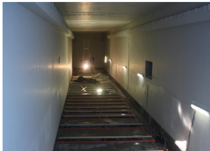
Linac tunnel preparation
