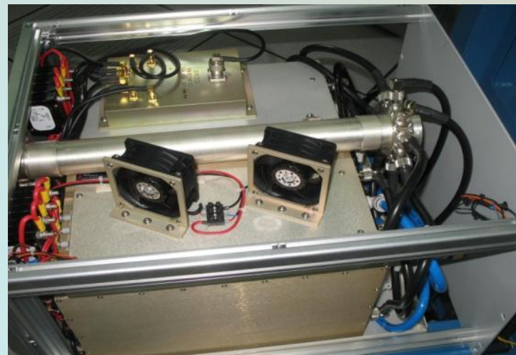
Inside view of the 5.5 kW drawer
