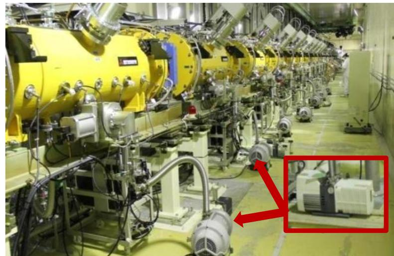
Oil rotary pumps are replaced with scroll pumps<sup>41</sup>
