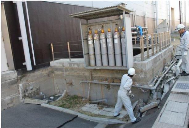
Figure 2: Subsidence near the entrance of the linac building. Water supply and drainage pipes were broken.
