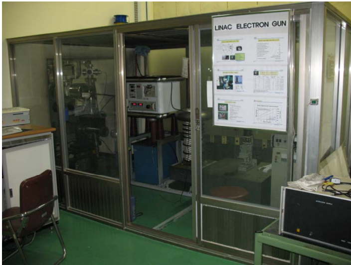
[Old Control room(Tunnel)]
