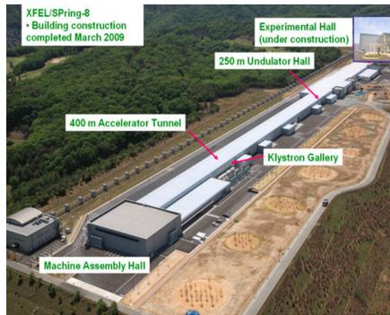
Figure 7: XFEL project at SPRING-8 construction status
