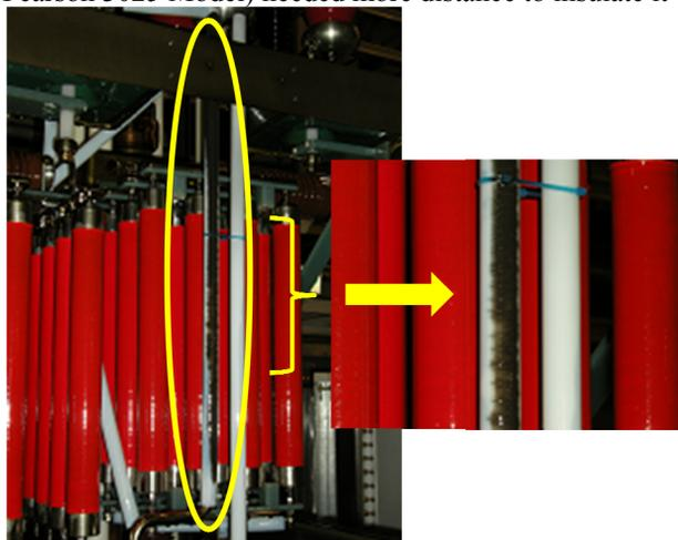
Figure5: Discharge traces in anode-modulator oil tank (in Area-1 of Figure 2).
